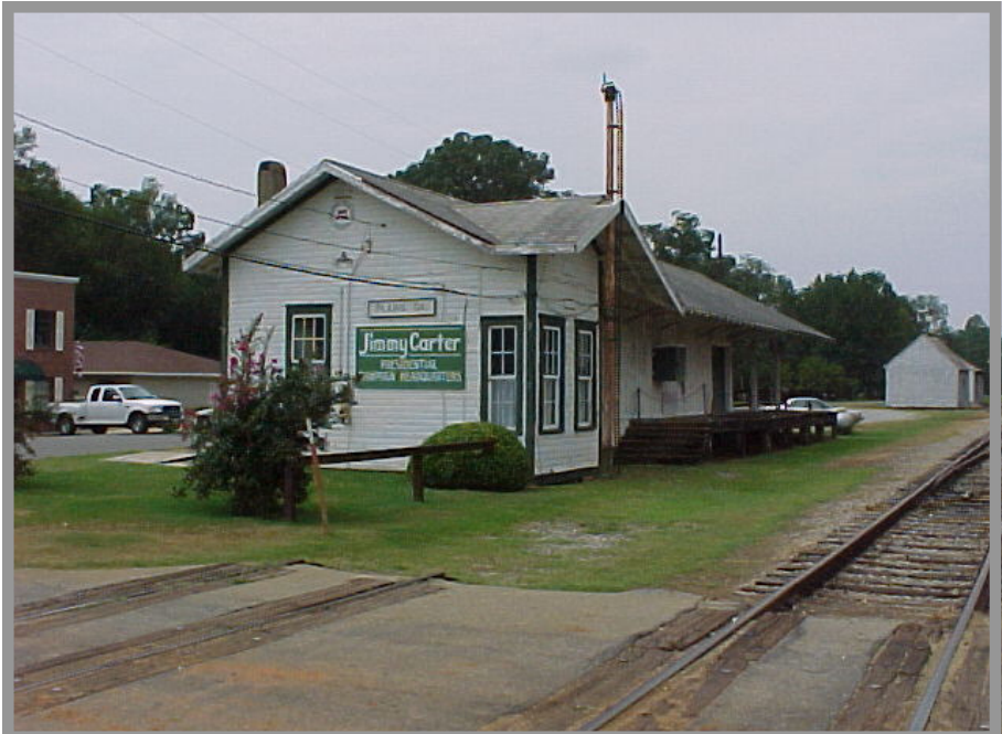
The exSCL depot in Plains, GA that served as the symbolic campaign headquarters for the Jimmy Carter Presidential effort. The building now serves as a part of the Carter historical exhibits in Plains. Digital image taken on August 31, 2001 by Chuck
